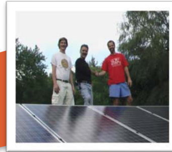
#5 Install Solar / PV
